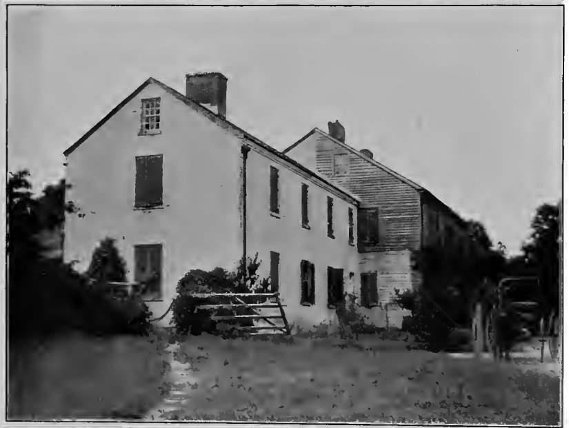
CLARENS HOUSE HOSPITAL.
