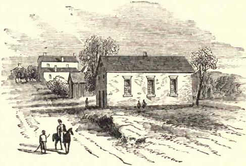
STONE CHURCH AT CENTREVILLE, VIRGINIA.
