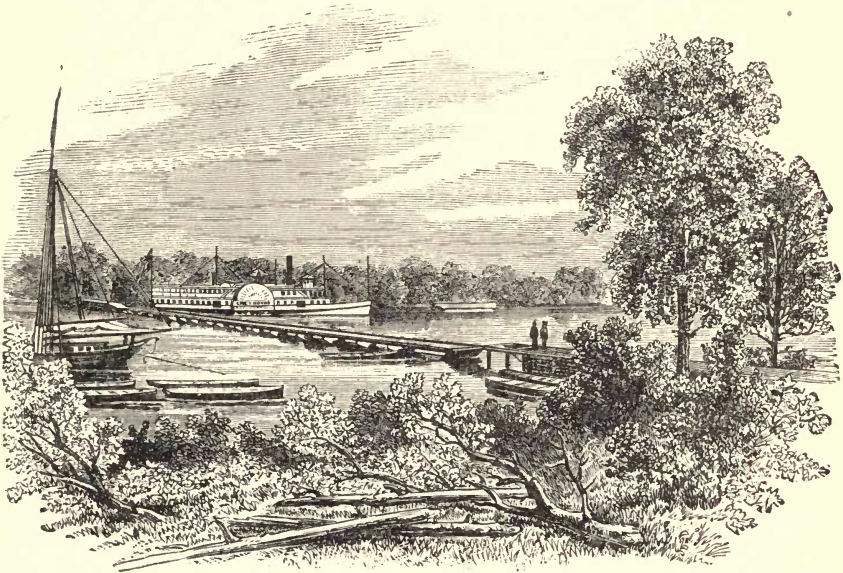
PONTON BRIDGE AT DEEP BOTTOM.
