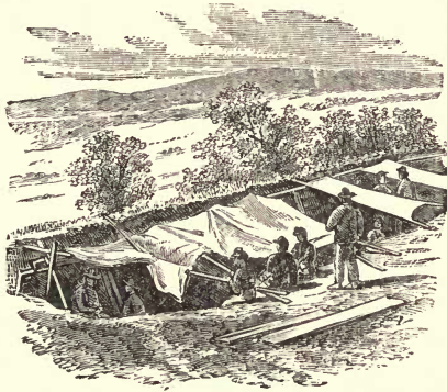
BEHIND THE EARTHWORKS.
