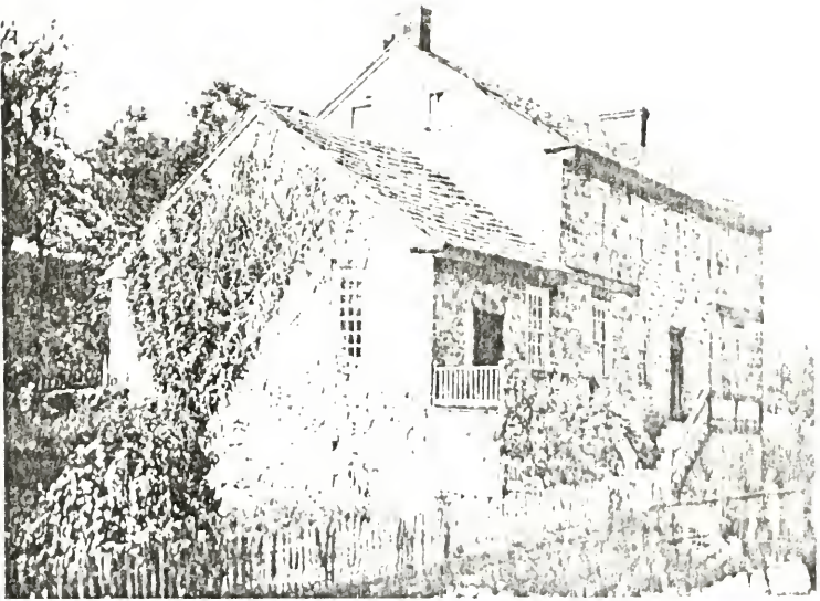
ROXBURY, JOHN SCHAFER'S HOMESTEAD, ERECTED 1782.
