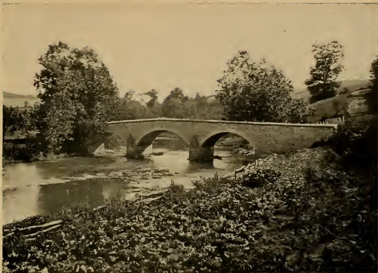
BURNSIDE BRIDGE AS IT APPEARS TO-DAY
