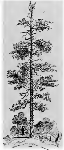
REYNOLDS'S STATION, S. E. of Atlanta.
