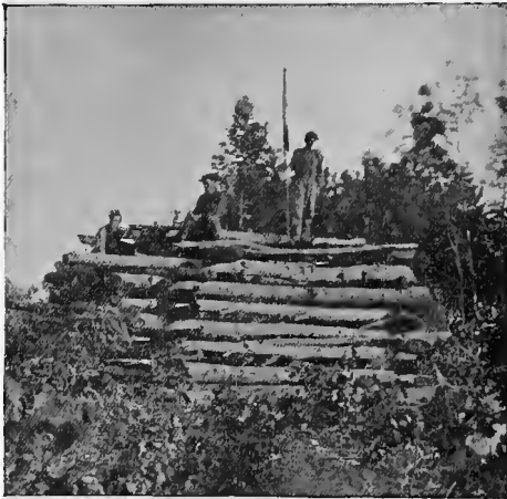
ELK MOUNTAIN STATION, OVERLOOKING ANTIETAM.
