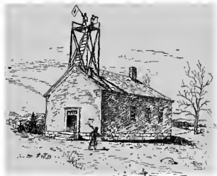
STATION ON PARISH CHURCH, YORKTOWN.
