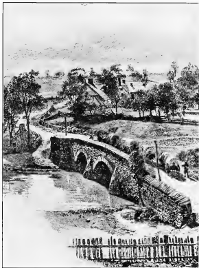
Orndorff Mill Bridge Over the Antietam.
