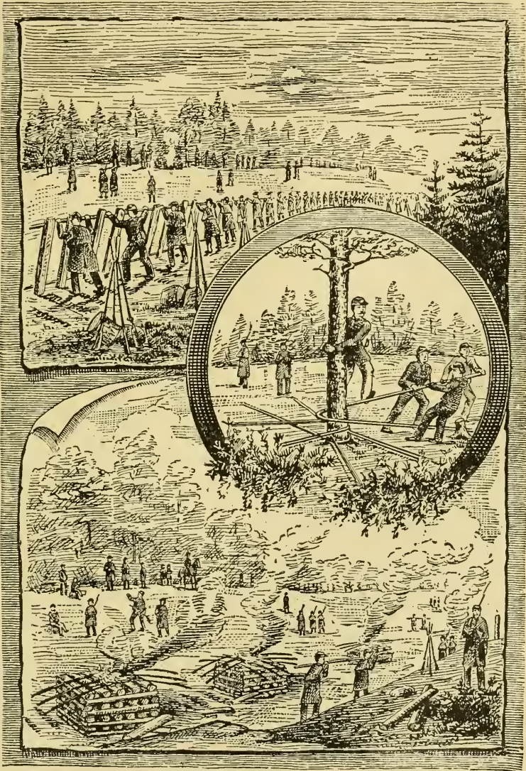
TEARING UP THE WELDON RAILROAD.
