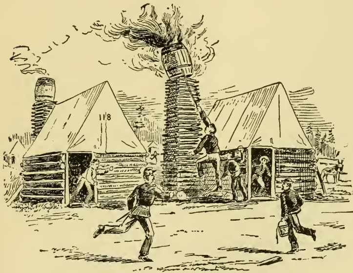
FIRE! FIRE! TOTAL LOSS—NO INSURANCE.
