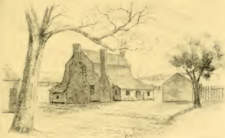
Jarvis Farm Hospital
