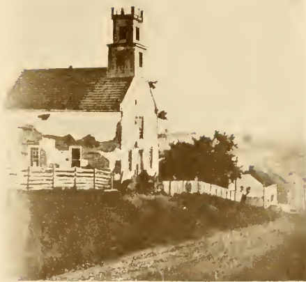
LUTHERAN CHURCH IN SHARPSBURG, EXTERIOR WAS HARD PLASTER FINISH, DAMAGED BY ARTILLERY FIRING.
